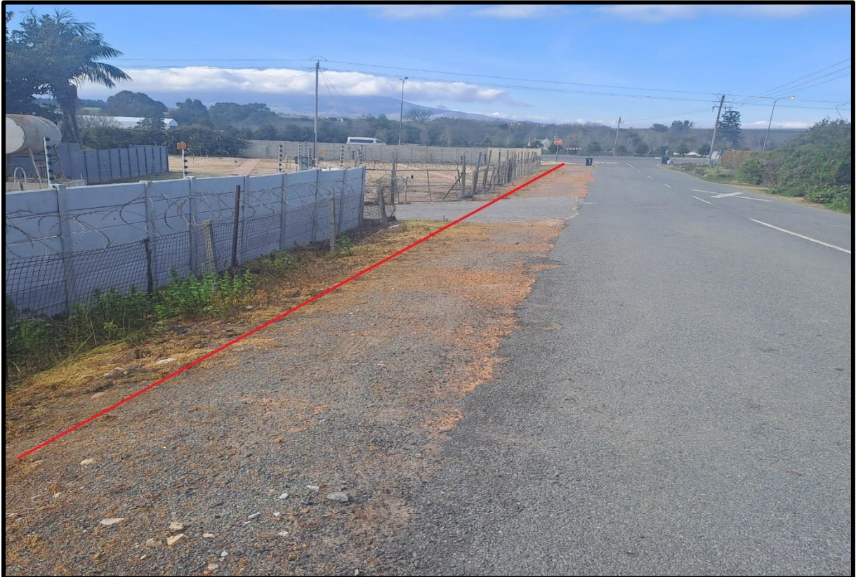
Fig 6: Underground cable route in the Vlaeberg Rd Reserve. View towards the intersection with Baden Powell Rd. Totally devoid of vegetation.
