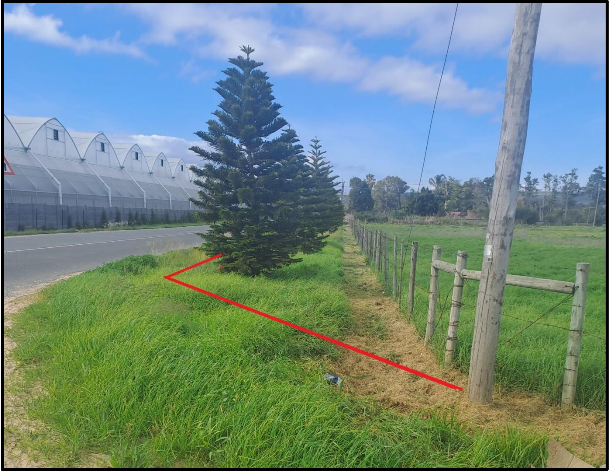
Fig 3: View of cable route from termination pole to edge of Vlaeberg Rd. Vegetation is mainly Kikuyu grass
