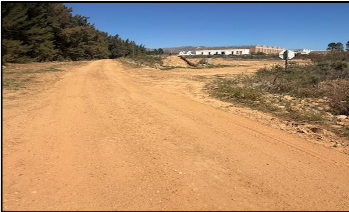
Figure 2: View of the route of underground cable where it deviates to the right to aim for the building.
