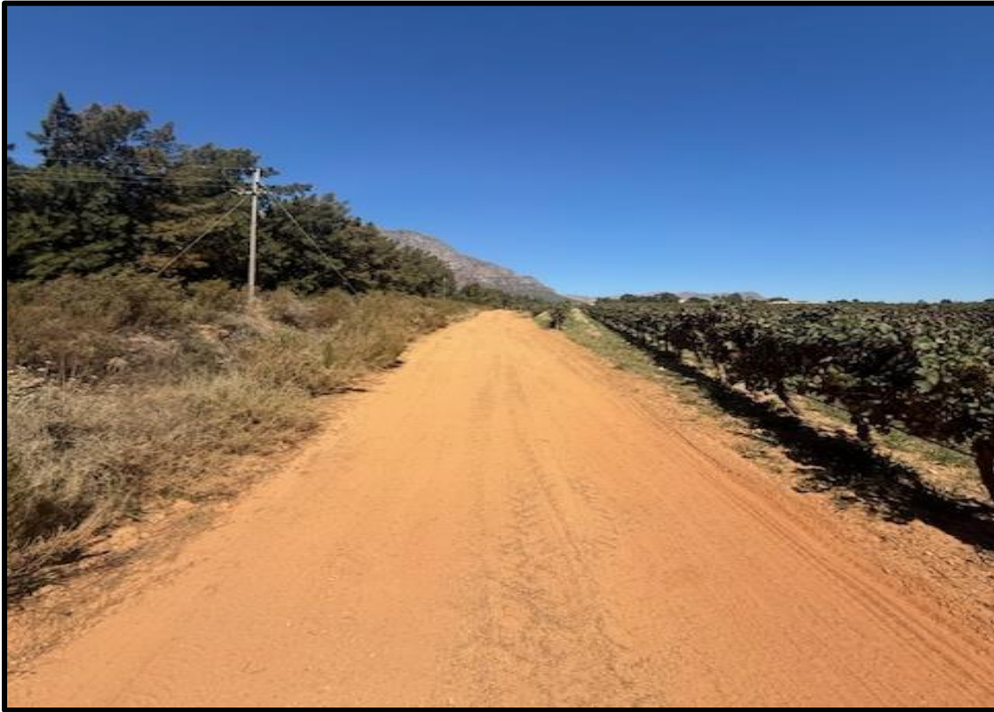
Figure 1: View of route of underground cable. Entrenched on the right edge of the road. Note existing overhead line on left. To be removed.
