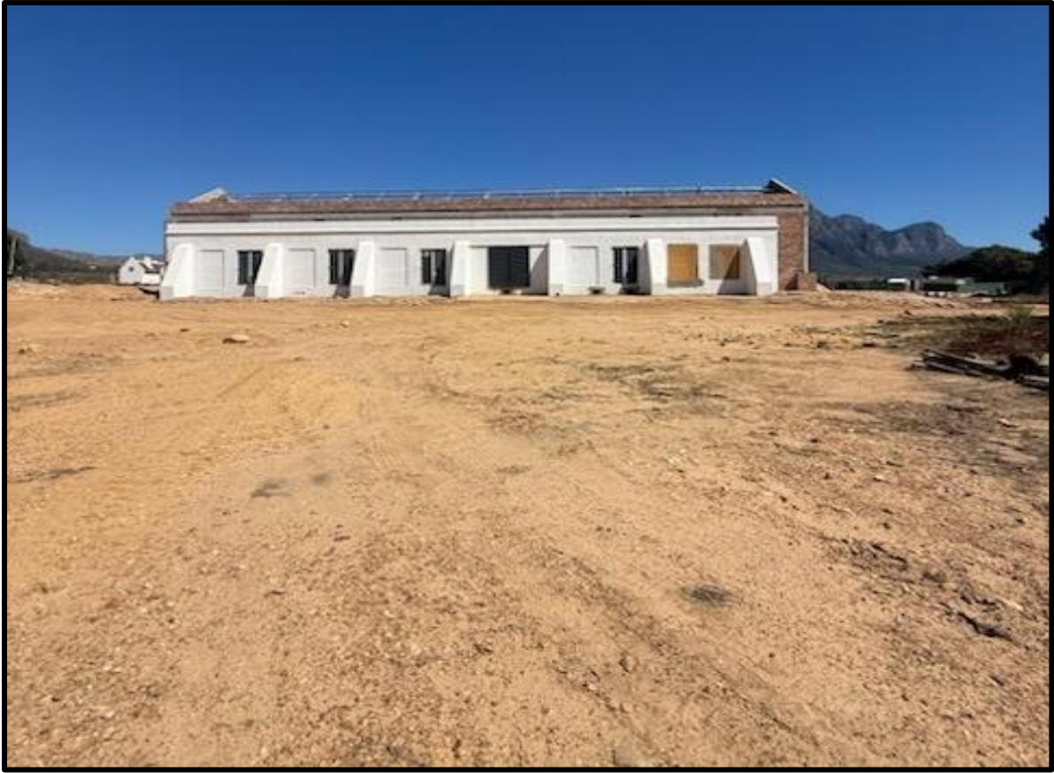
Figure 3: View of route of underground cable towards the righthand corner of the building.
